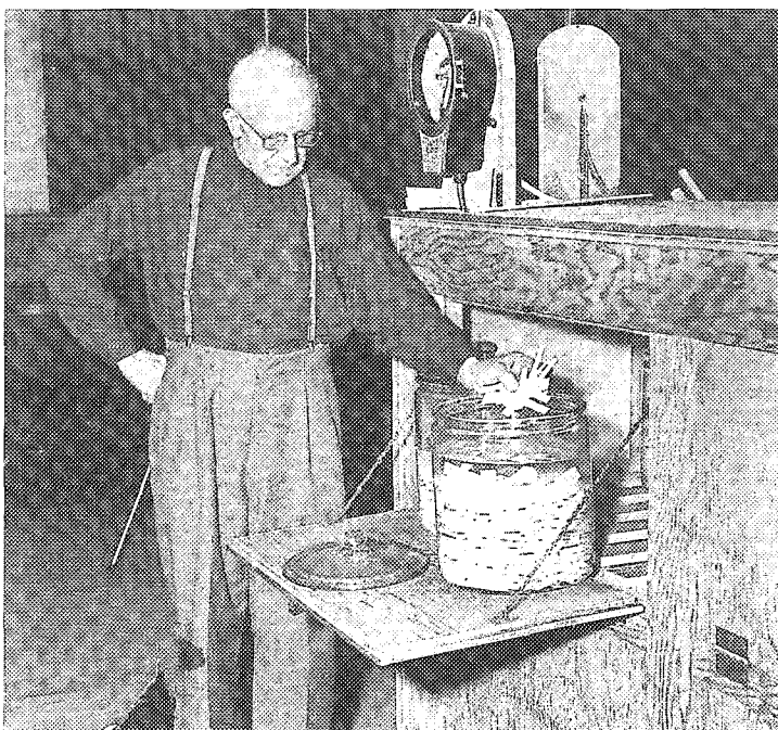
Figure 10. Wood & Brooks shop foreman Andrew Probst pulls a fistful of heads and tails from a jar of peroxide bleach, 1920s. Note temperature recorder and shrouded bleaching cabinet. Wood & Brooks Collection.
